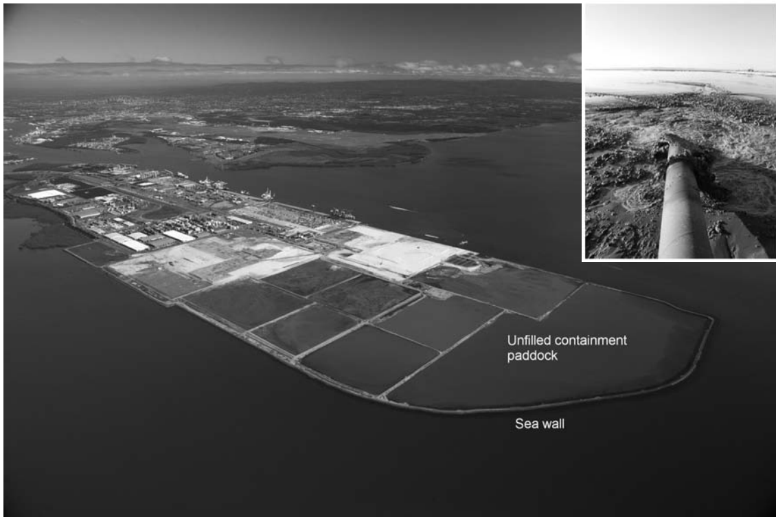
Figure 1.1 Land reclamation containment paddocks (Inset: Dredge spoil pumped into the containment paddock) (Courtesy of N. Sivakugan, James Cook University, Australia)
